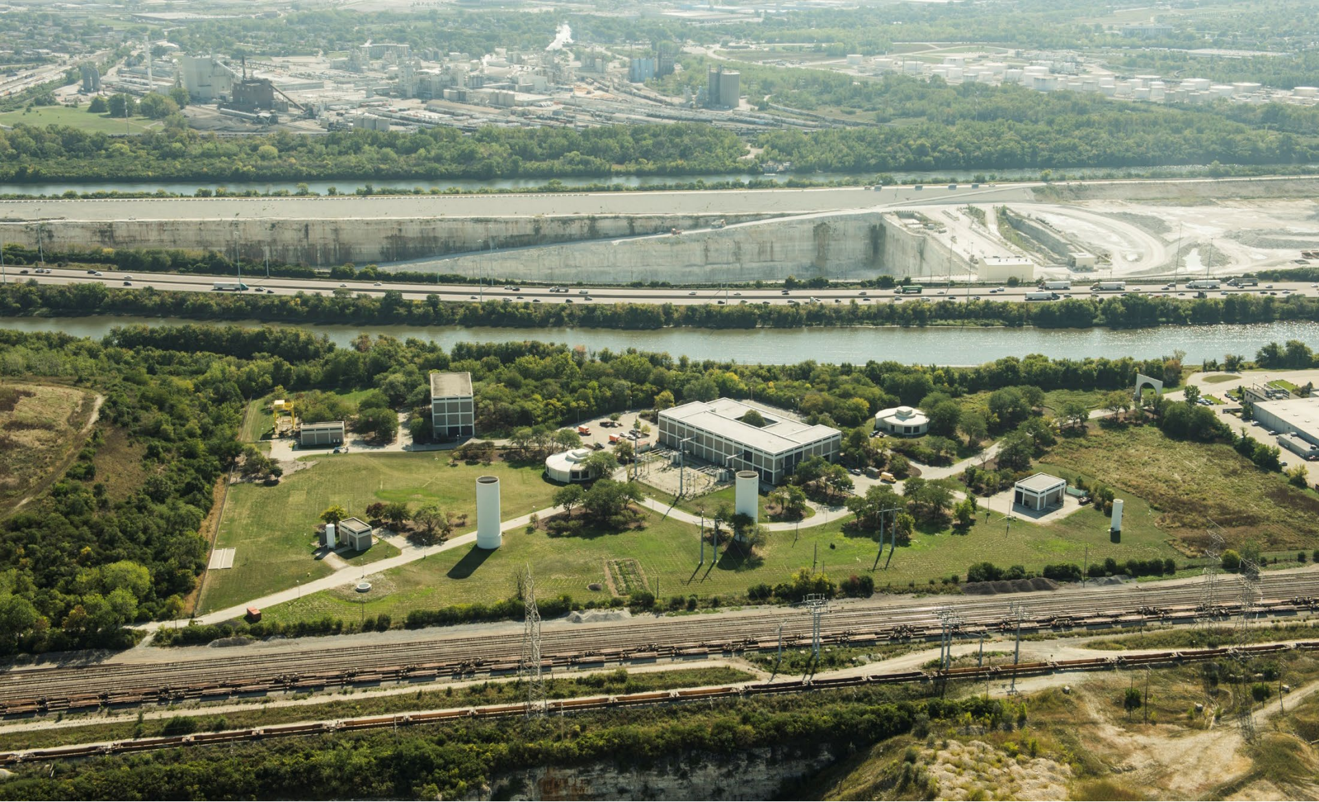
Mainstream Pumping Station
