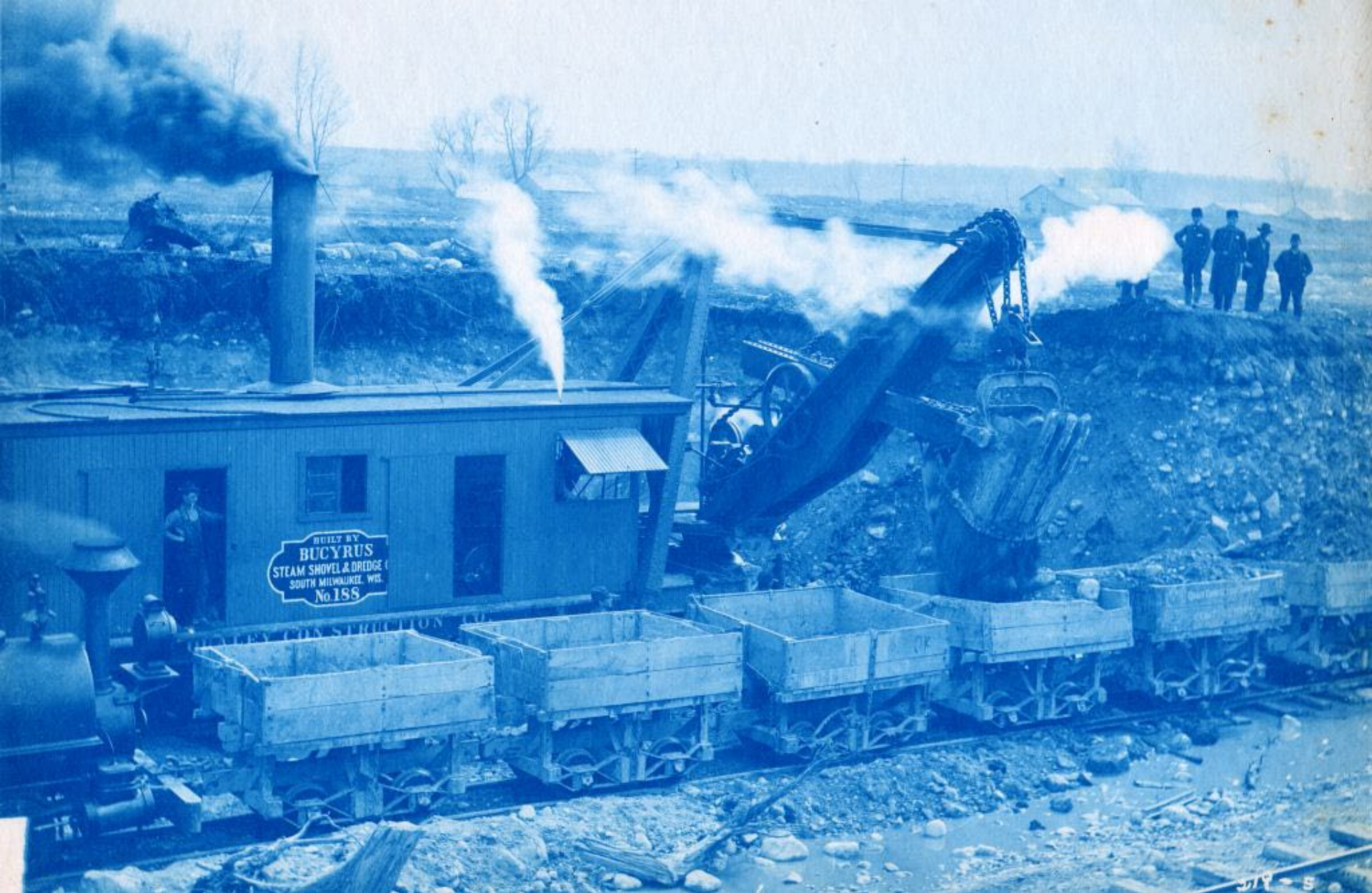
Steam Shovel Excavating Overburden 1894
